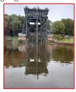
we went to the Anderton Boat Lift. This is one of only two working boat lifts in the UK. It is known as the Cathedral of the Canals. It was designed to do the lifting of boats and barges 50 feet from the River Weaver Navigation to the Trent and Mersey
